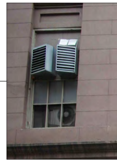
EXISTING VENTS TO BE REMOVED
