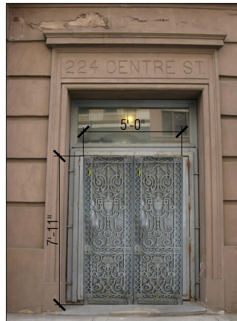
SUPER IMPOSED PROPOSED CAST IRON DOORS ON EXISTING BUILDING
