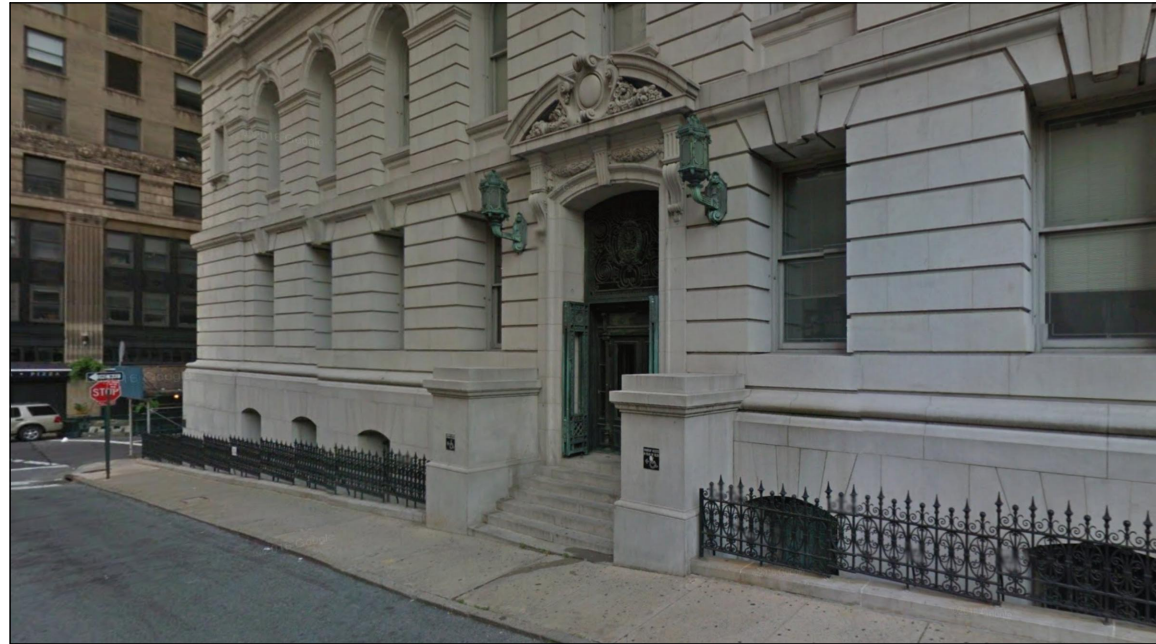
NYC MUNICIPAL LIBRARY - 1 ELK STREET ENTRANCE
